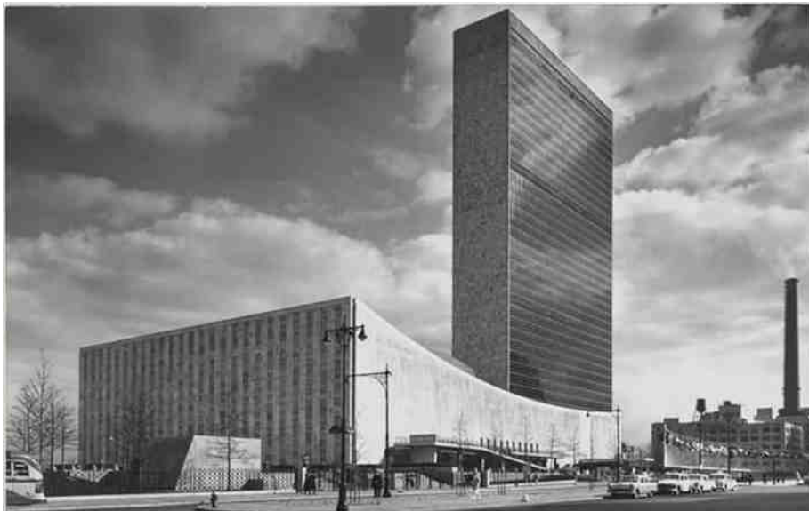
Figure 4: United nations headquarters (168 meters) with its glass facades [Image courtesy: ny.curbed.com ]
