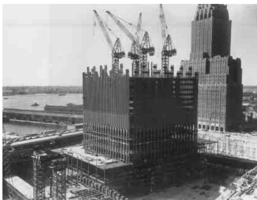
Figure 5: Construction of erstwhile world trade center using four Kangaroo cranes [Image courtesy: raredelights.com]
